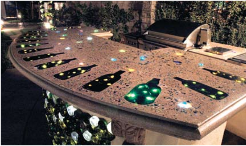
Combining crushed, recycled glass with cast concrete, Scott Cohen of The Green Scene creates one-of-a-kind polished “stone” surfaces for outdoor bars and kitchen areas. The resulting surface can be backlit for dramatic illumination. Photo courtesy of The Green Scene .
